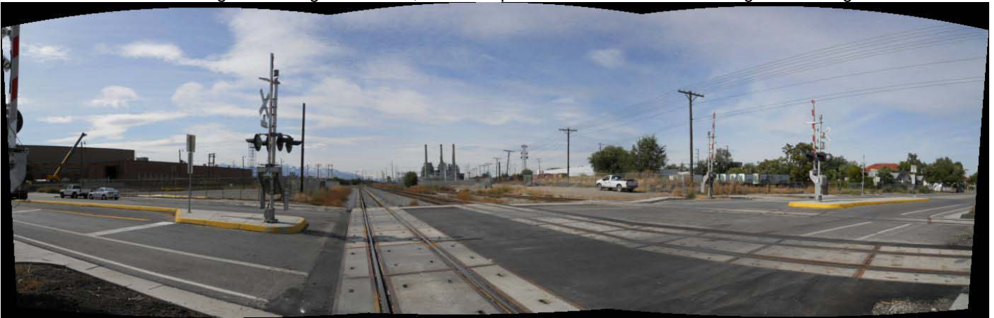
Panoramic view - looking west along UP rail line; Undeveloped Folsom Avenue runs along the building shown at left
